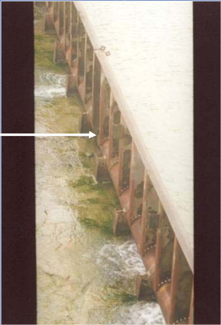
Bolted connection at gate's field splice
