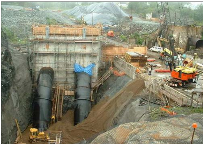
Construction of intake and penstocks
