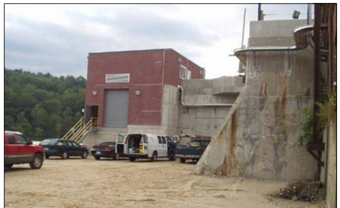
Exterior of new powerhouse nearing completion
