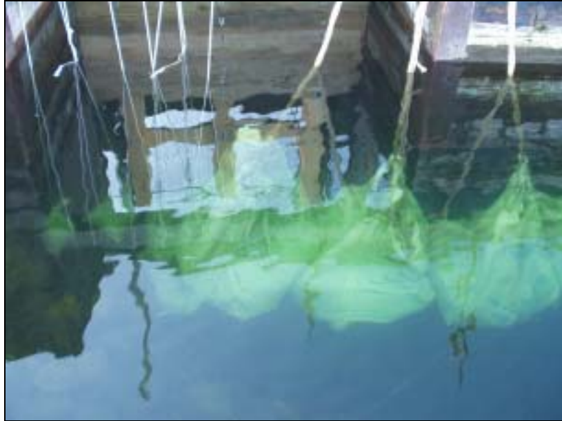
Sandbags Filling Voids Upstream of Gate Apron
