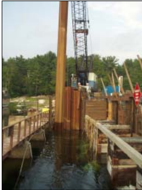
Installation of Phase I Cofferdam against Eastern Abutment
